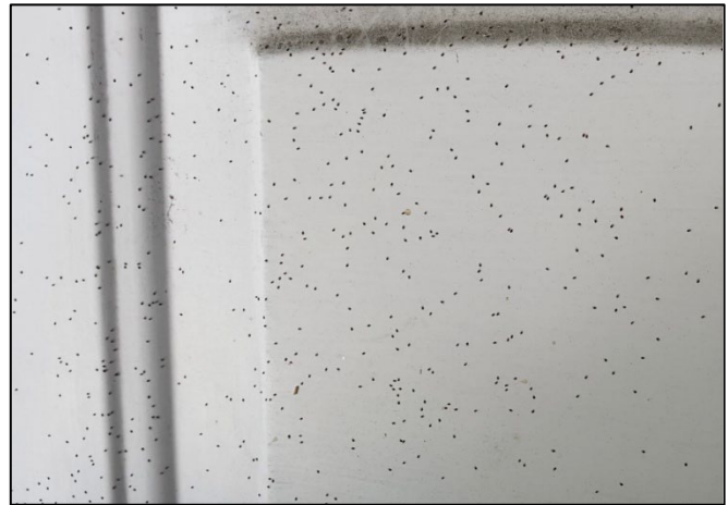
Bird mites covering a front door after dispersing from an abandoned bird nest on a front porch.
