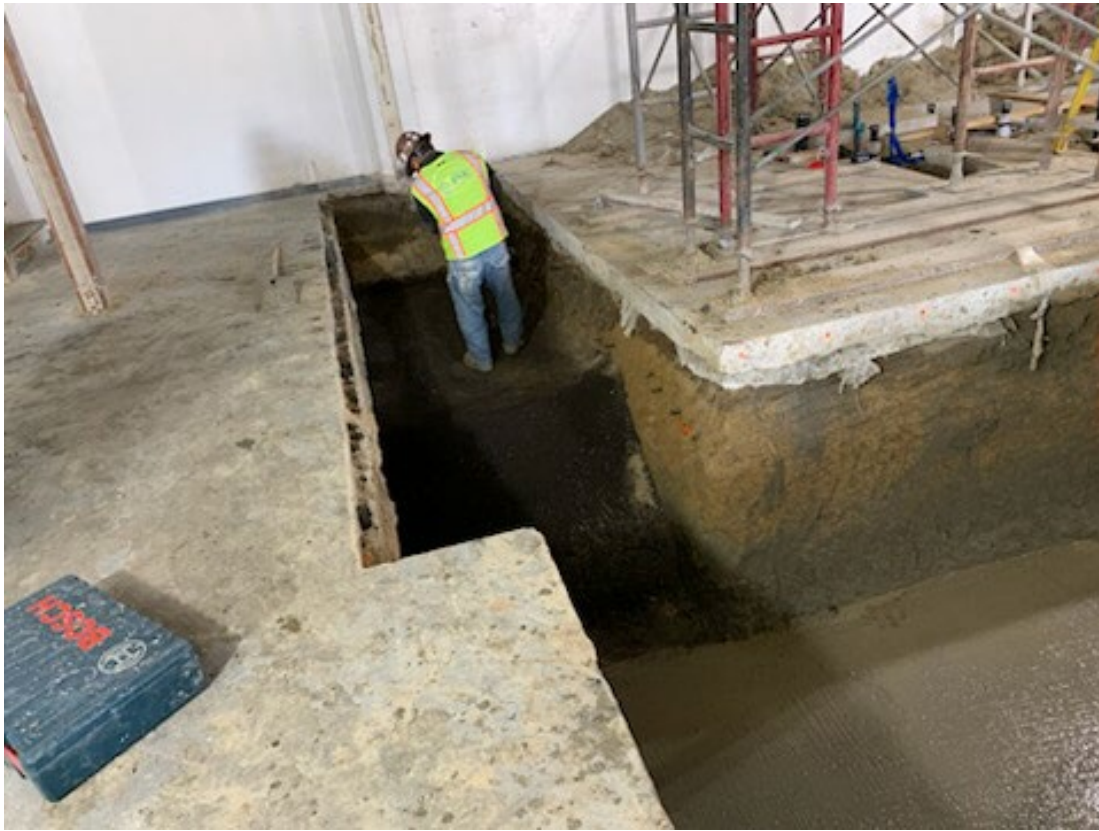
Elevator Room and Pit Foundation
