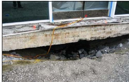
Construction opened an entry point under the foundation
