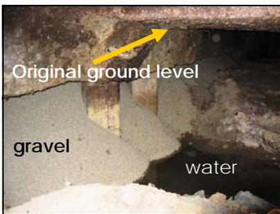
Void created under foundation by subsidence. Original ground level was flush with foundation (arrow). Note gravel on left (placed to seal out mosquitoes) and standing water (lower right)
