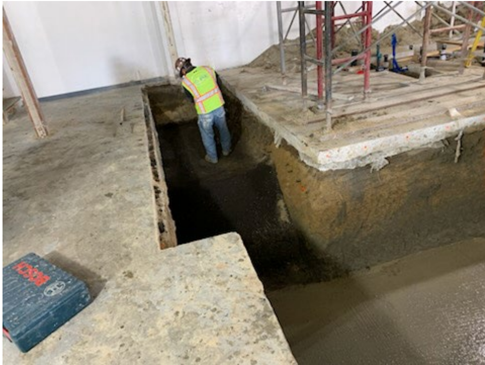
Elevator Room and Pit Foundation
