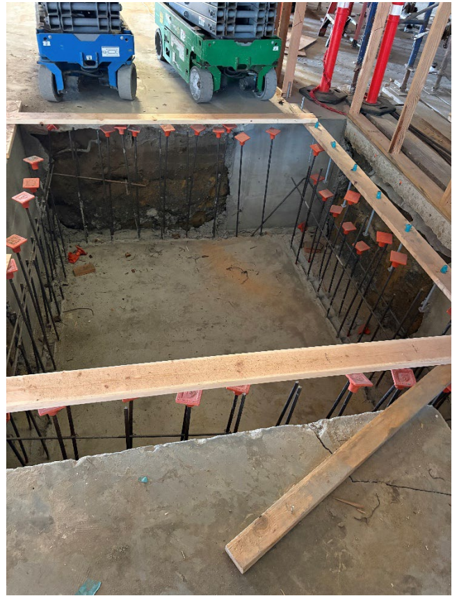
Base of elevator shaft
