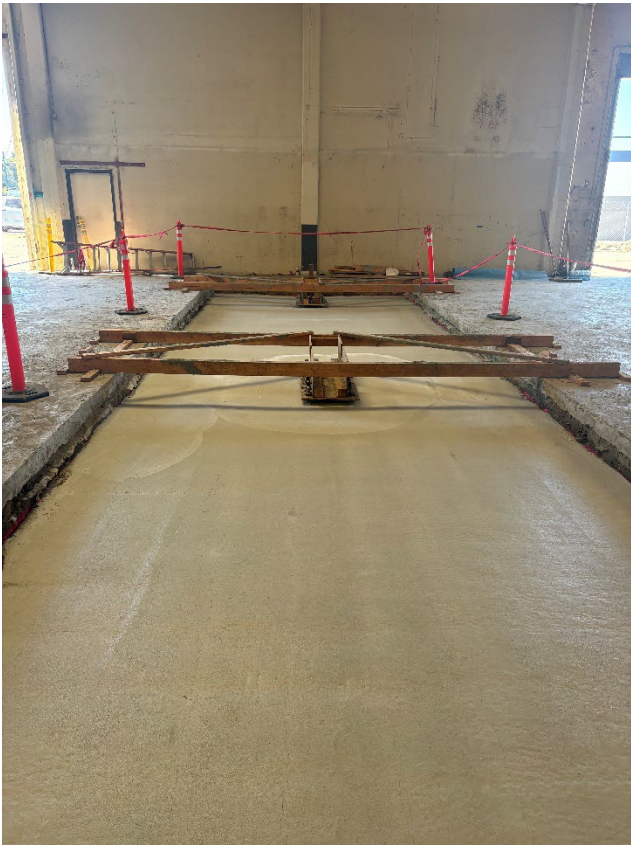
Spread Footing for large earthquake retrofit shear wall
