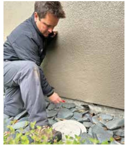
Operations Director Casey uses a small mirror to check for a gap where rodents might enter along the bottom edge of a wall.
