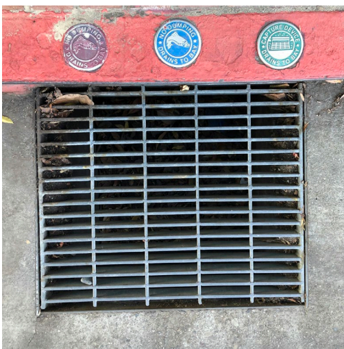
This storm drain has circular markers to indicate that it drains to the Bay.
