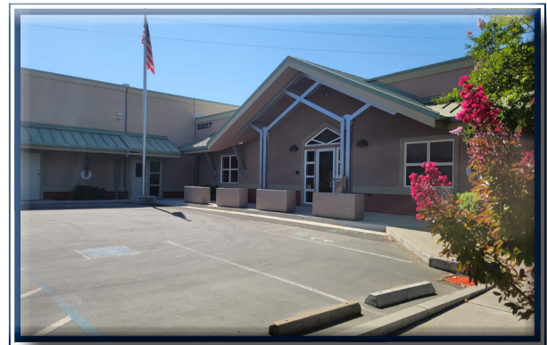
SOUTH PLACER MUD RENOVATED ADMINISTRATION BUILDING
