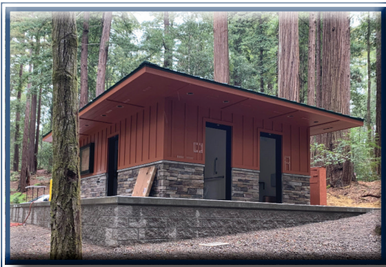
NEW RESTROOM BUILDING
